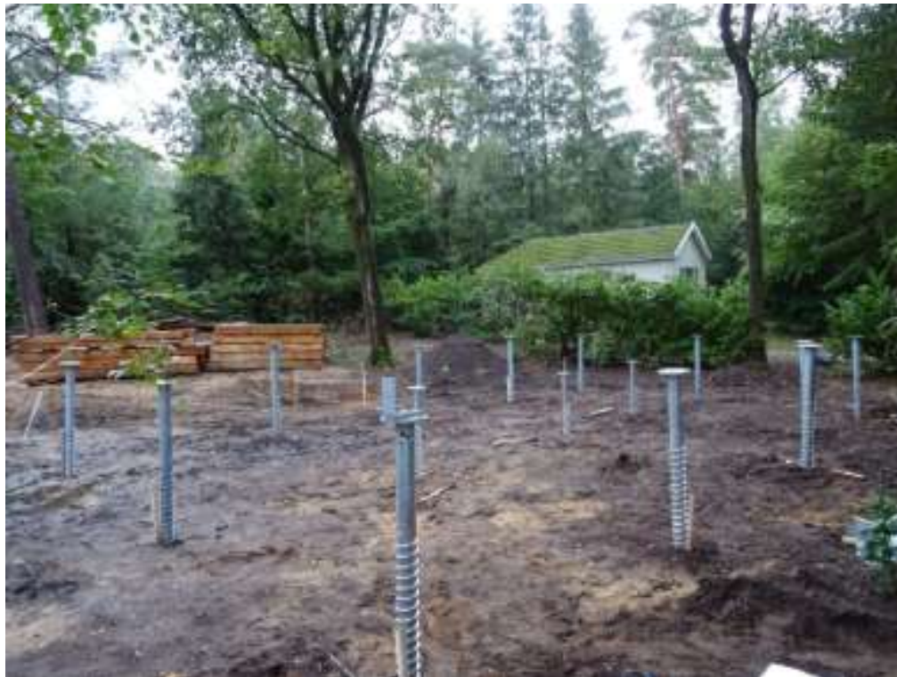
Figure 1: Example of ground screw foundation system.
